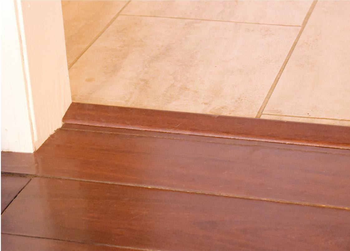
Our floor transition has been just laying on top of the floor for about a year now, and is easily kicked out of place on accident all the time! The wood flooring transition comes with a little track that the transition snaps into. The tile flooring in my kitchen is taller than the living room wood floors, so the space in between is too deep for the track to reach! Our solution? RapidFuse to the rescue!
